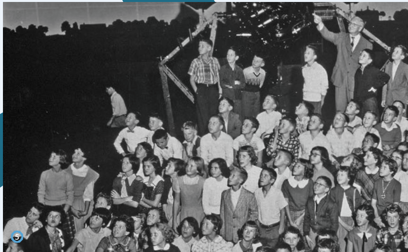
1 John Motley Morehead III (center) with Coach Bob Fetzer (left) and John Lindsay Morehead II (right) 2 John Motley Morehead III 3 Construction of the Morehead Planetarium Building, 1948 4 The new Morehead Planetarium Building in the snow, as seen from Franklin Street 5 Children visit the new Morehead Planetarium 6 Family members Julie Newton and Motley Morehead at the laying of the Morehead Planetarium cornerstone; Motley (daughter of John Lindsay Morehead) later became the first female trustee of the Foundation 7 The finished Morehead Planetarium was the first of its kind at a public university 8 The Zeiss Planetarium Mark II Model Projector, 1949 9 John Motley Morehead III places items in the time capsule to be embedded in the cornerstone of the new Morehead Building
